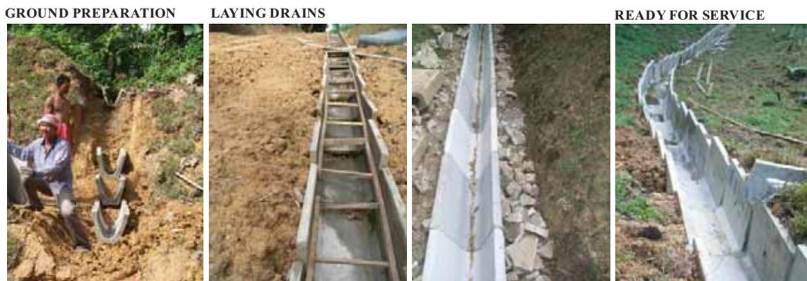
**Figure 9:** Unsupervised drainage work on extremely loose dumped soils. Where drains are replaced, old drain are broken up and used as fill. (Gasing hill entrance 2008, July)
