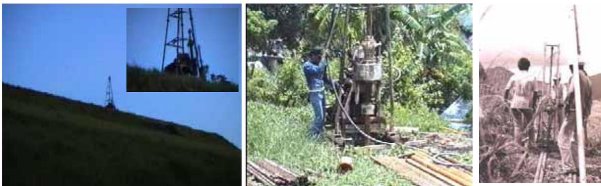
**Figure 2:** First two photographs on left show boring rigs used almost everywhere. These rigs use are not acceptable as “water jetting” method is used to advance the hole. Acceptable sample of a light rotary boring rig is shown on far left. Actions of both these rigs are described in Figure 3.
