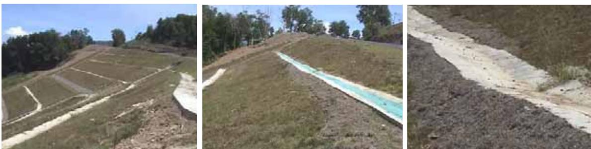
**Figure 7:** Cast in place drains are already experiencing settlement while this slope is still under construction
