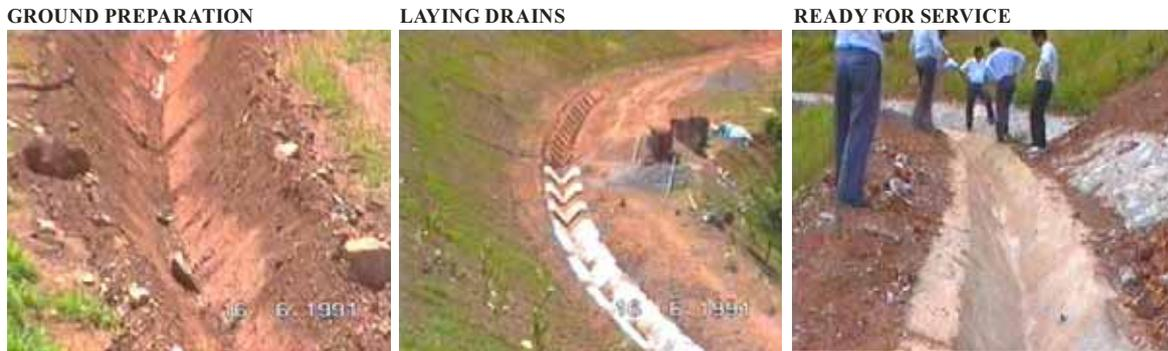
**Figure 8:** Good ground preparation, alignment and construction of drains (East West Highway 1991)
