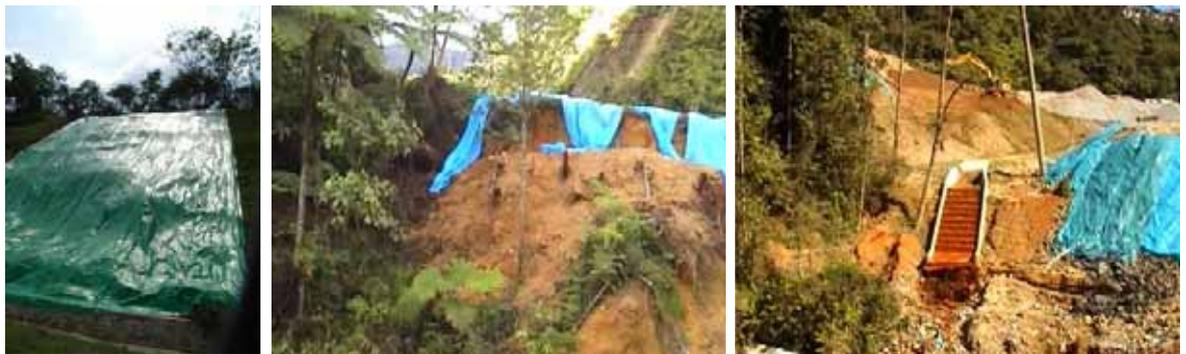
**Figure 16 :** Covering slope against rain, only the slope on far left is an example of proper cover, rest just pretending.
