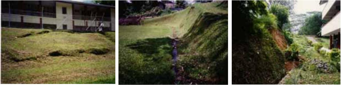
**Figure 14 :** Institutional slopes in various stages of distresses from ground movement to toe drains silted over or blocked
