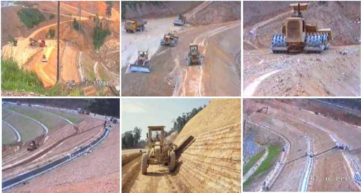
**Figure 5:** Well executed slope construction with down up construction. Neat, well compacted and trimmed slope faces. (East-West Highway)
