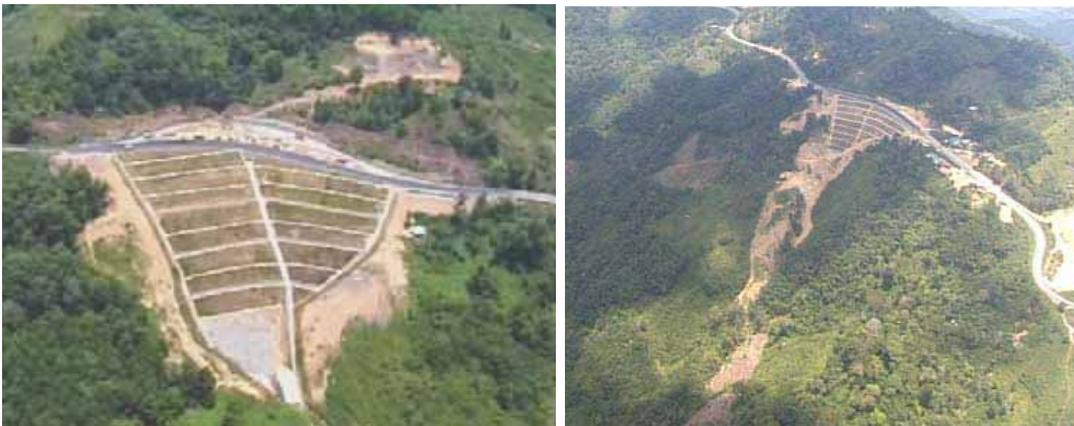
**Figure 4:** Slopes seen from close up and from distance. Illustrating problems of safety for maintenance crew. Narrow berm widths and lack of measures against falling over makes sites like these impossible to maintain. Designs have to address such issues.
