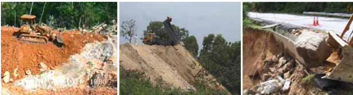
**Figure 6:** Building up slope by dumping soils and waste down slope. Discarding rock-fall debris down the slope on the other side
