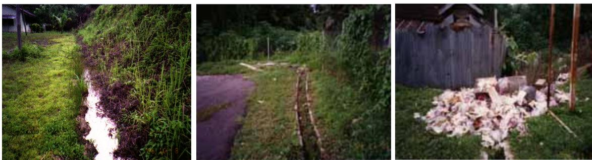
**Figure 13:** Damaged drains deteriorated to ditches, drains clogged up, drains used as rubbish dump. This one is just above a steep slope.
