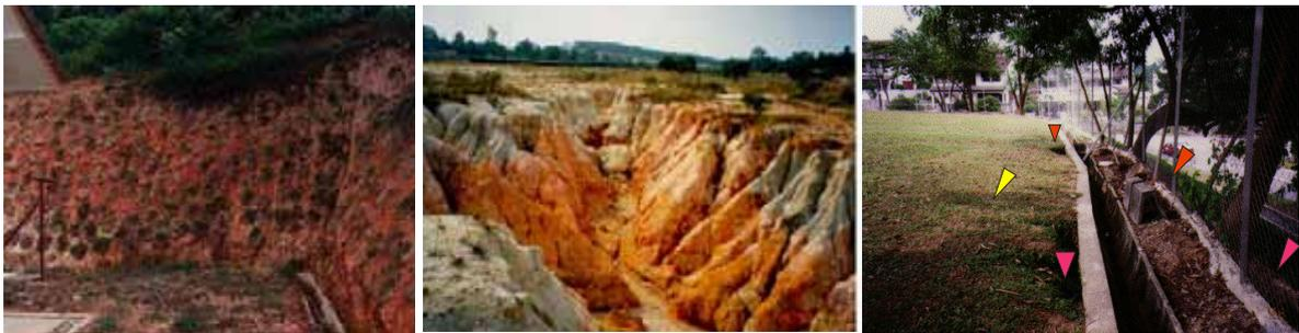
**Figure 15 :** Spot turfing going bad, erosion gullies as deep as 5 meters and cutoff drain above slope with number of “sinkholes” developing
