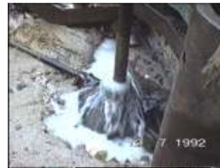
A\_Rod with adapters attached to NMLC core barrel about 30 meters down inducing fractures into cores due to whipping
